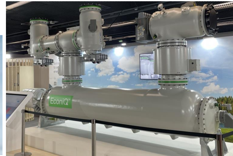
Hitachi Energy 420 kV C4-FN / O 2 / CO 2
