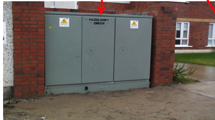
MV/LV Substation
