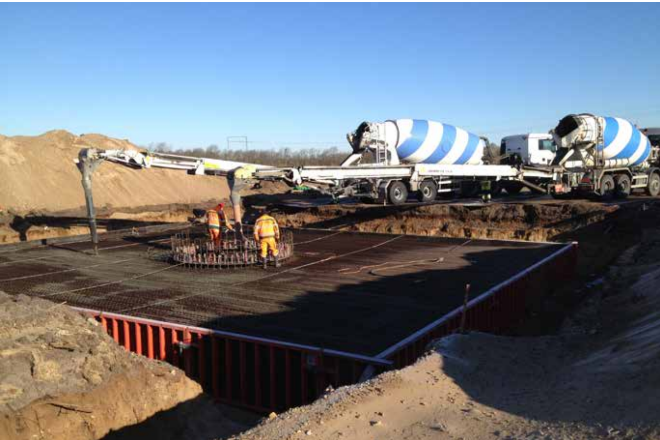
Lattice Tower foundation ( 21 days )
